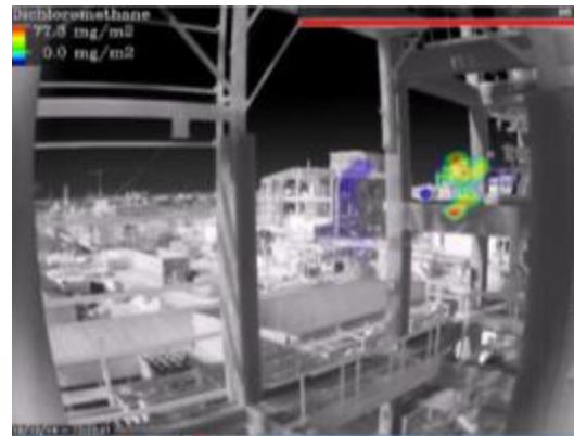
2: The Second Sight has detected 1 leakage at 250m.
