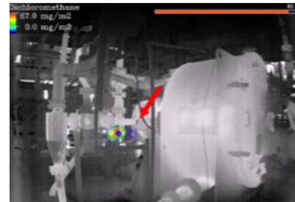
3: The Second Sight has detected a leakage at 5 meters while the operator is identifying the source point with thermal imaging (black point).
