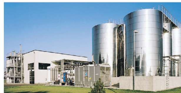
ecoMotion Biofuel Plant in Malchin, Germany
