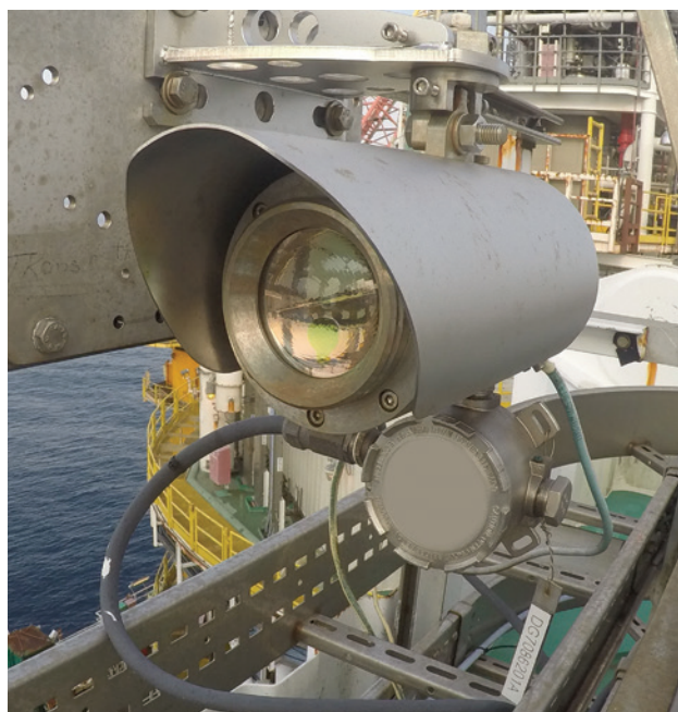
Figure 2: Senscient ELDS laser-based open path gas detector
