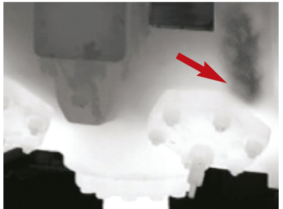
Inspectahire has been using thermal imaging cameras for a long time to detect dangerous gas leaks.
