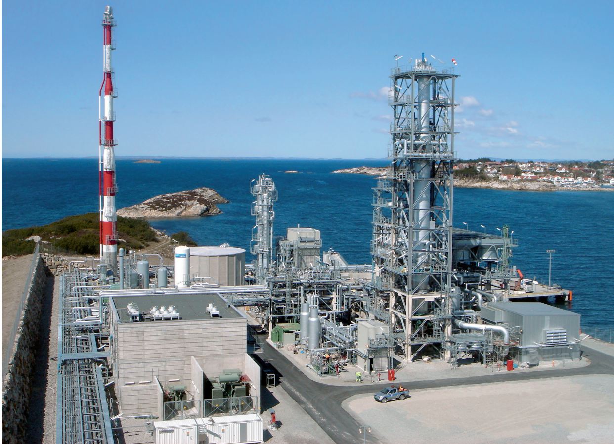
Figure 1: LNG is the big trend: Linde is building a medium-sized natural gas liquefaction plant with a capacity of 1.5 million tonnes of LNG near the Russian Baltic Sea town of Portovaya (Symbolfoto; Linde AG).
