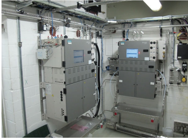
Picture 3: System integration: Analyzer house with 2 process GCs - Optimized for best reliability using liquid sample streams
