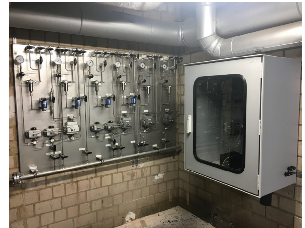
Picture 4: Sampling system design variants for liquid samples – heated in cabinet (right) and unheated on SS plates (left)
