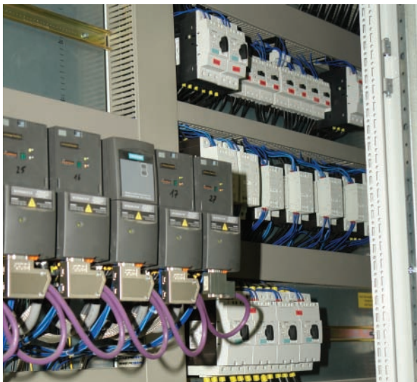
Figure 5. For drives with varying speeds, the Micromaster MM440 by Siemens has proven a rugged "all-rounder" which offers particular ease of handling.
