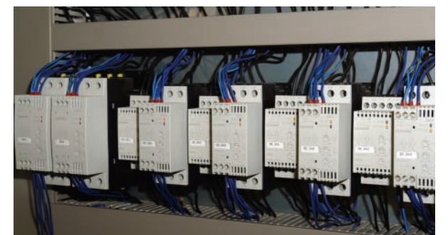
Figure 7. Start-up time and voltage as well as ramp-down time can be comfortably set for the 3RW30 soft starters via potentiometers.
