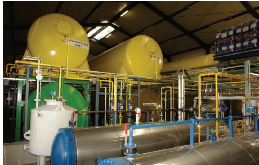
Figure1A and figure 1B. In the Kassel biodiesel production plant, all important sensor and actuator signals are transmitted to the central control station via Profibus.
