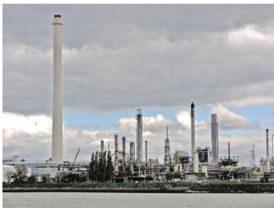
Figure 1: A large site with refinery and petrochemical facilities
