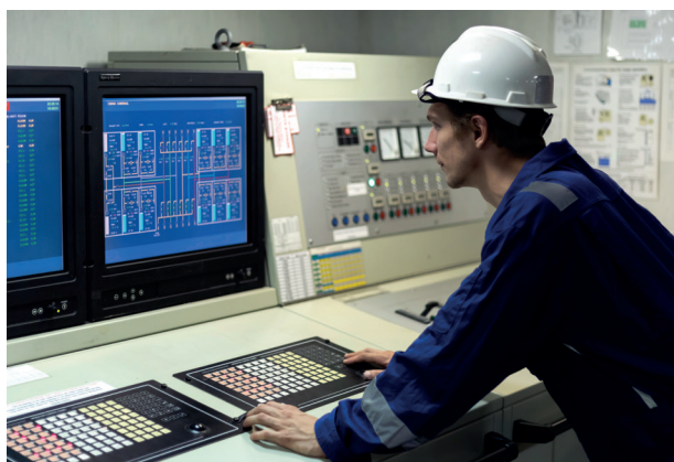
Cargo hold monitoring system
