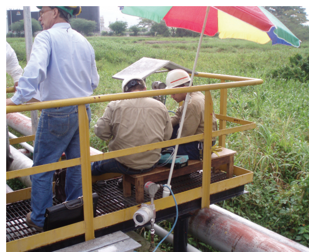
In-Situ calibration of DP cell
