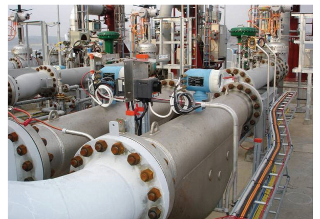
Modern inlet mass meters used for fiscal applications
