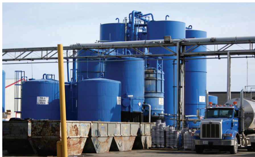
Newalta measures the level of oil in 19 recycling tanks with 18 Echomax XPS-30 transducers connected to three Sitrans LU10s.
