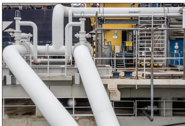
Measuring point on jetty 1 (above the framework set up for installation)
