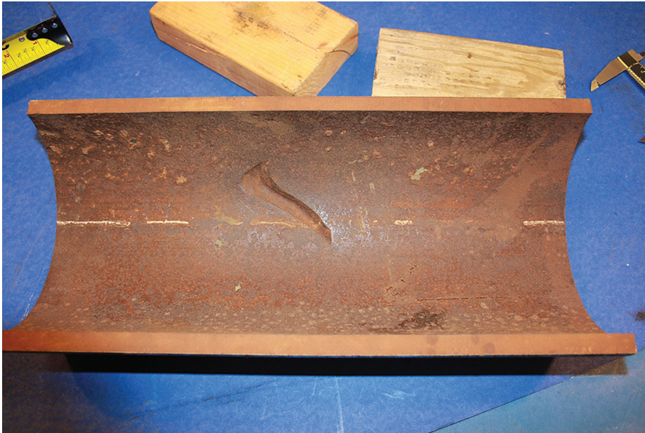
Manufacturing defect in seamless pipe
