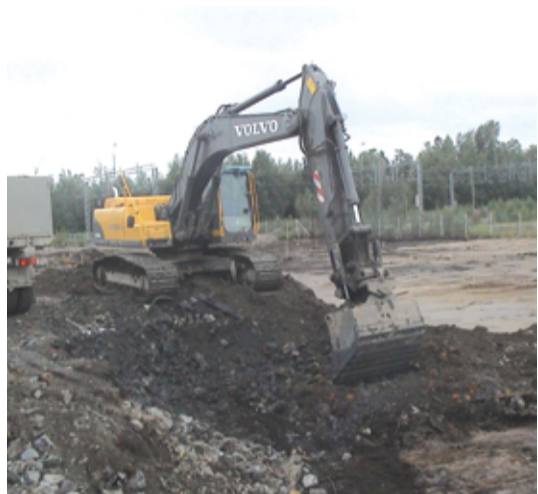
Figure 6. Contaminated soil removal
