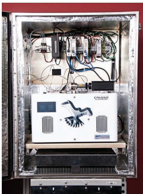
A Calidus GC installed in a typical process enclosure.
