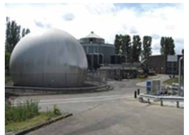
South West Water's Countess Wear Sewage Treatment
